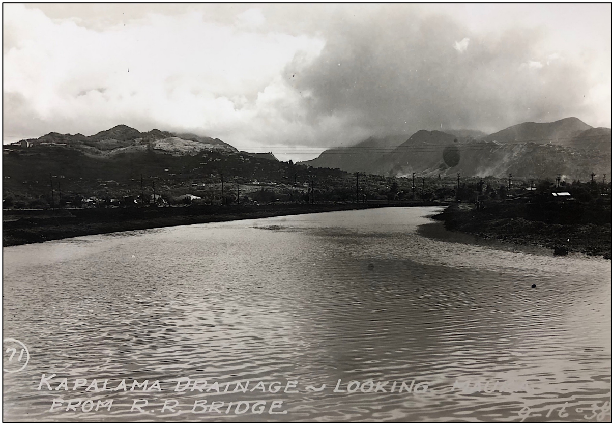
Figure 30. 1938 photo of Kapālama drainage looking mauka from R.R. Bridge (Bishop Museum Archives SP20711,3)
